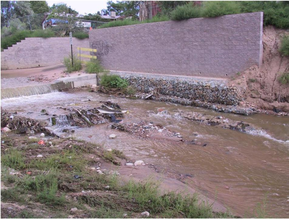
Photopoint 2, looking upstream at retaining wall under construction. August 30, 2006. Note that loosely placed fill is gone and dirt covering footings of gabions is gone. Also note graffiti.
